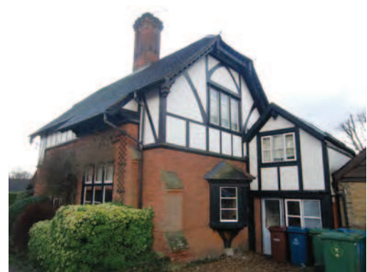
Picture 1.35 View looking south towards 47 West Drive
