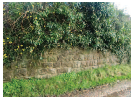
Picture 1.60 Dry stone wall along the top of West Drive
