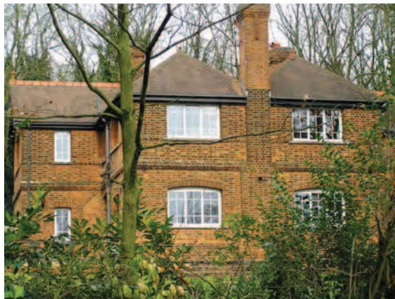
Picture 1.8 3&4 The City, Old Redding before a recent fire which part destroyed the building
