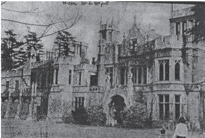
Picture 1.11 Early 20th century photograph of the mansion. Source: Harrow Observer 1980.
