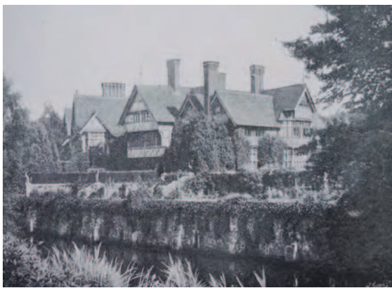
Picture 1.11 Grim's Dyke Hotel 1891
