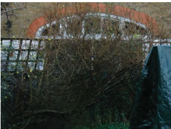
Picture 1.28 Central gauged red brick arch
