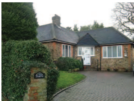
Picture 1.50 51 West Drive
