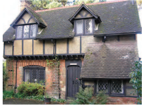
Picture 1.39 North Lodge LBH LA.100019206.2013
