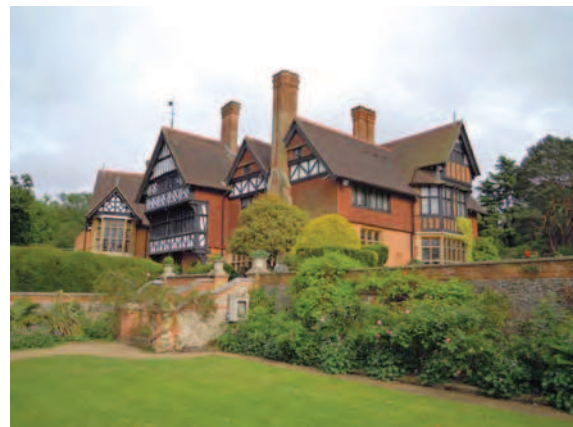
Picture 1.12 Grim's Dyke Hotel 2013
