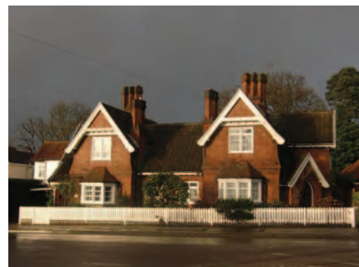
Picture 1.48 148 and 150 Uxbridge Road (former Gamekeeper's lodge)
