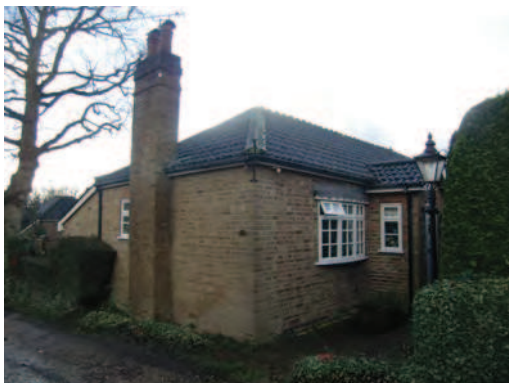
Picture 1.41 42 West Drive
