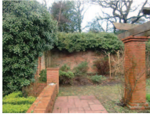
Picture 1.35 18th century brick walls to formal garden at the Kin, Brookshill with 20th century additions to the front
