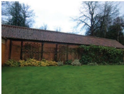
Picture 1.34 Replica drying sheds within the Kiln site, Brookshill re-using original clay pantiles
