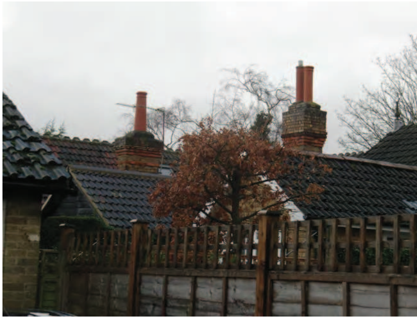
Picture 1.21 Good view towards chimneys and pots of numbers 40-44 West Drive from just outside the Conservation Area
