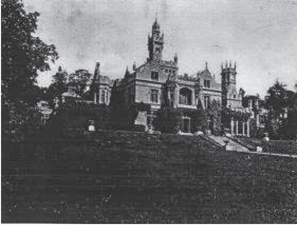
Picture 1.9 19th century photograph of the former mansion house with slope in front part of the landscaping - still in place. Source: local history library.
